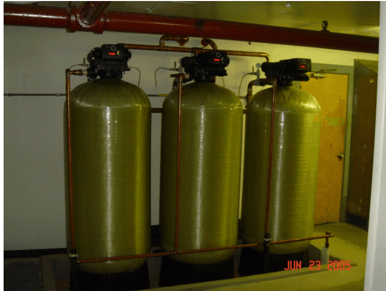
Argentine Convalescent Center MEDIA G2 PLANT
